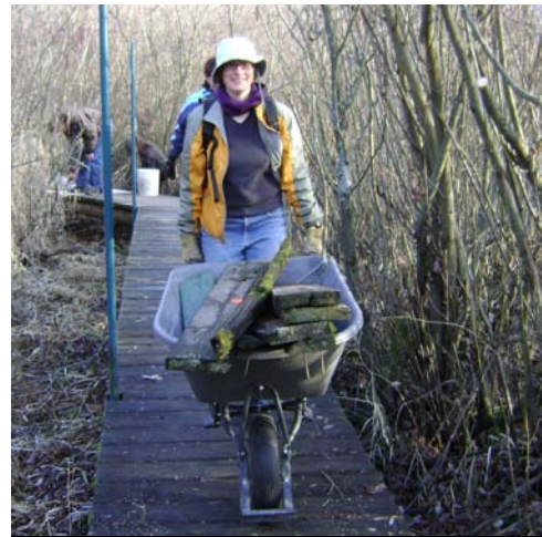
Volunteers complete repairs to Waldie Trail boardwalks in 2008.
